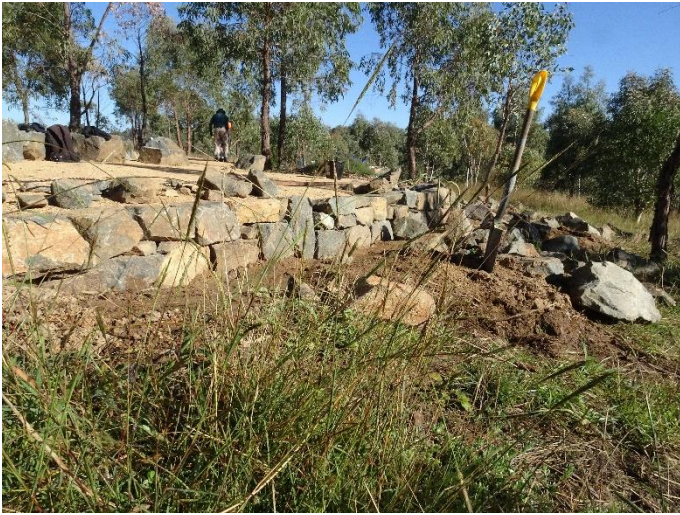
We are building a low rock wall to protect a path edge near the new entrance.
